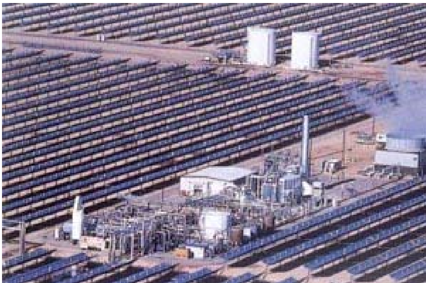
Figure 9. View of SEGS trough based solar thermal power plant in southern California.
