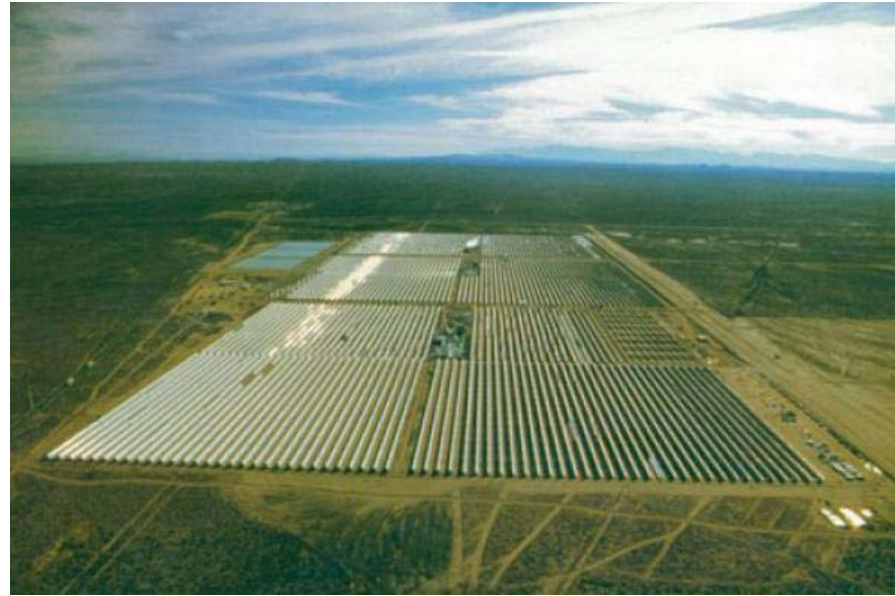
Aerial photo of existing 310 MWe SEGS Power Generating System in California's Mojave Desert
