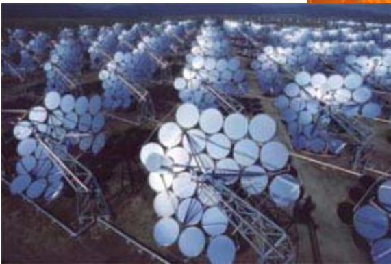
Figure 12. Solar Plant 1, 700 dishes producing steam.
